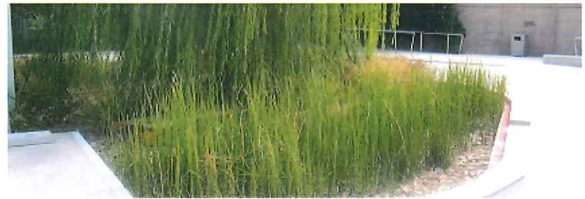
Figure 8: Curbs with openings or breaks permit the redirection of stormwater into natural planted areas. (Photo Credit: EPA)
