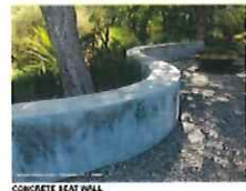
CONCRETE SEAT WALL
